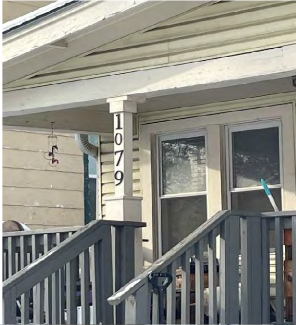
1079 Western Ave N Reinspection on 1/5/2026
